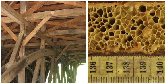
Figure 2: Two low density structures can be observed in the figure: (left) an example of a truss used in a bridge, and (right) an example of a honeycombed structure found in the Durvillaea antarctica alga (©Andre-Philippe Drapeau Picard)
