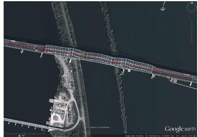
Figure 8: Linear overlaid on Google Earth ® Champlain bridge image.
