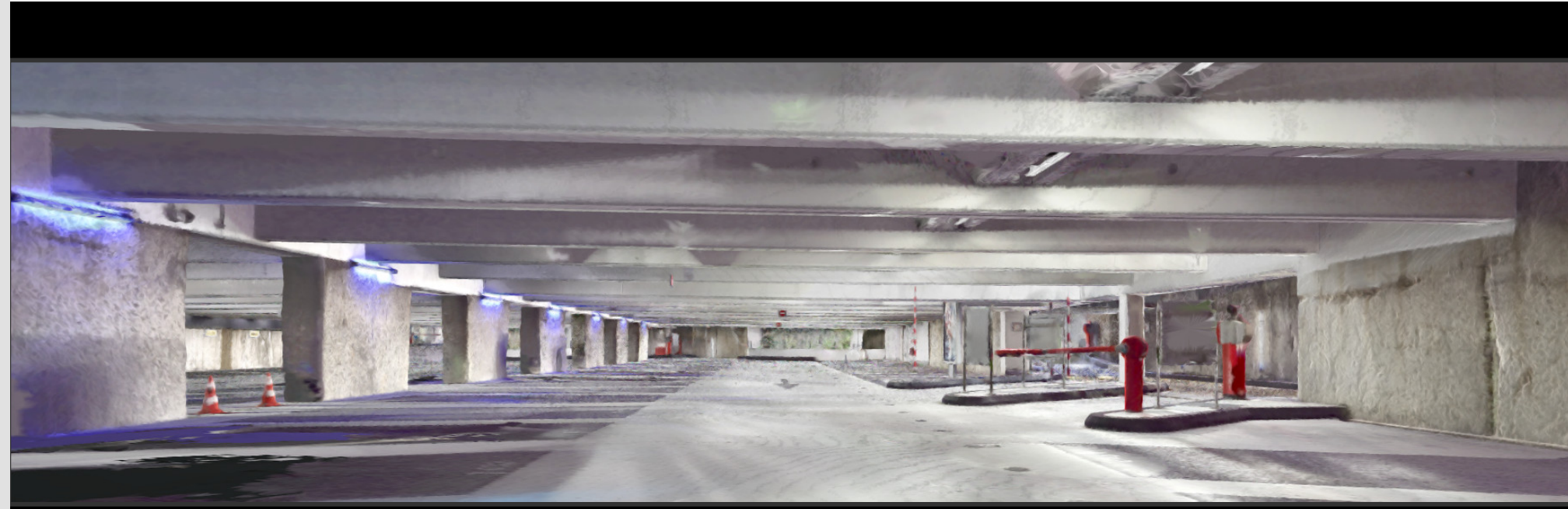
Figure 1: Underground Parking, provided by QPark
